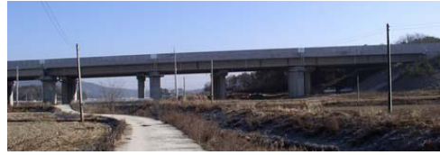
(b) Side view picture of the bridge.
